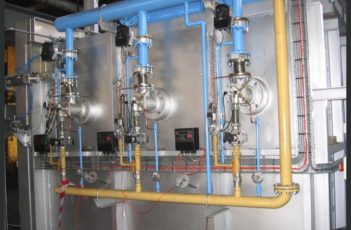
Fig. 2 Burners on reheating furnace.
